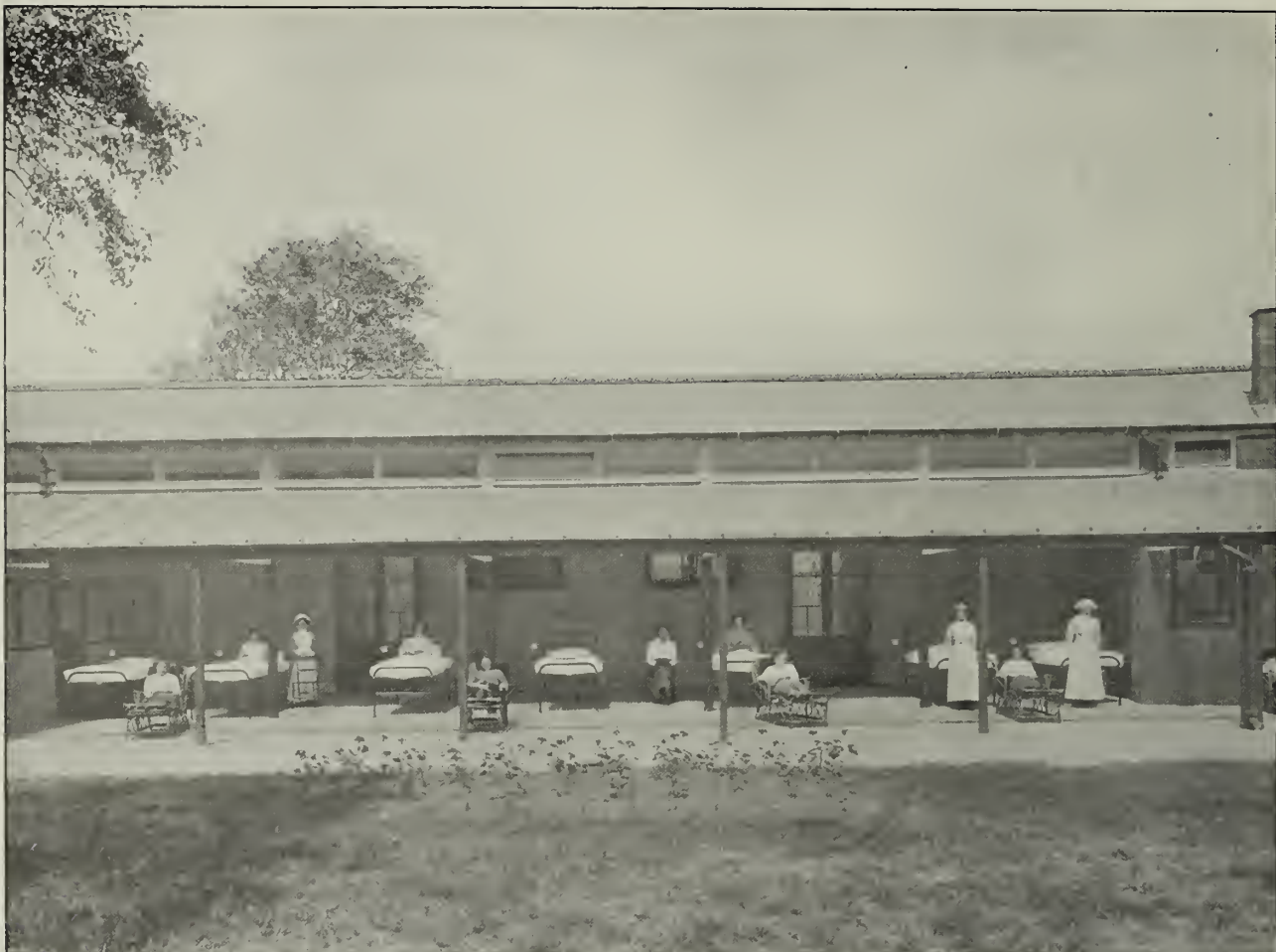
II.—Section of Yardley Road Sanatorium, where equally good results are obtained in the air of Birmingham. Note that the tuberculosis patients are treated in an open shed capable of giving protection from rain and snow only. There are comfortable dressing rooms immediately in the rear.
